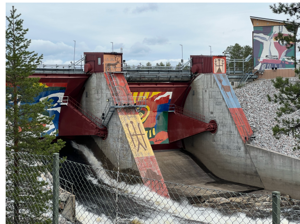
Fig. 1. A hydroelectric dam in the vicinity of Jokkmokk, Sweden.
