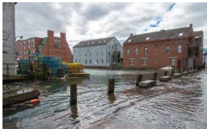
During the January 4, 2018 Nor'easter, powerful storm waves occurred at the same time as high tide. Water levels in Portland reached 13.8 feet, one of the three highest tides ever recorded. The tide remained above flood stage for nearly three hours, causing millions of dollars in damage statewide (Schmitt and Uteuova 2018).
