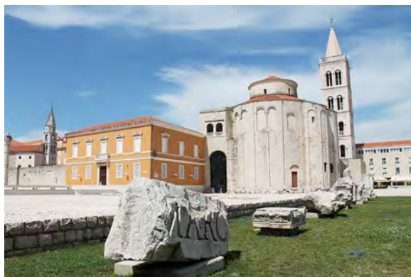
Fig. 1. Central Zadar with the 8 th century C.E. church of St. Donat (center-right) and fragments of the Roman forum from the 1 st century C.E.
